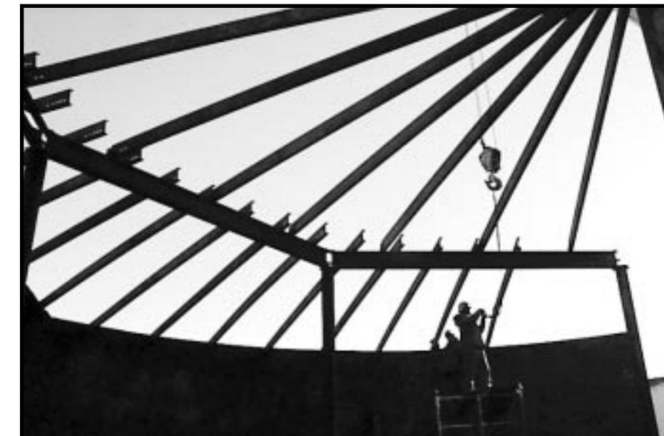
Tom Hopkins and Ross Dupuin battled with the winds as they dismantled the M2 fuel tank. "The wind picks up these sheets like a sail," said Dupuin. "You've got to be careful up there." Built in the 1950s, M2 is being taken off-line due to its age.
