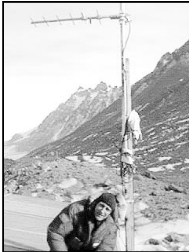
Robert Zook takes a break from working on a solar panel used to power the rural telephone system at Lake Hoare. The Yagi antenna above him transmits the signal to a repeater mounted on a ridge in the distance.
