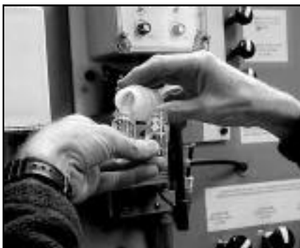
Allen Berggren tests the pH and chlorine levels of freshly desalinated waters inside McMurdo's water plant.
