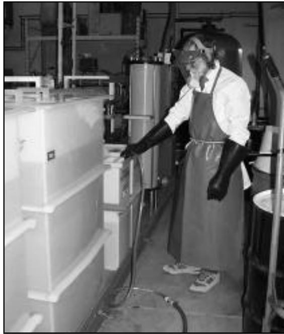
Water plant operator Al Berggren charges the hydrochloric acid tanks, a corrosive prevention measure that extends the life of the McMurdo water distribution system.
