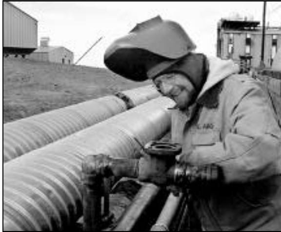
Patrick Stevens, a pipefitter, works on a fuel line that shares space with the new heat recovery system running between buildings 165 and 155 in McMurdo.
