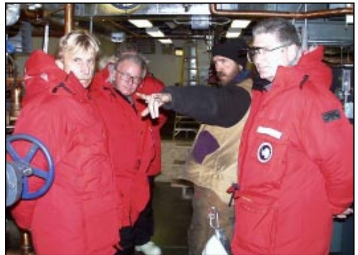
A 10 year veteran of the Antarctic program, Walker manages the construction crews at South Pole Station. "It looks nicer than most garages in the States," Hirsch said. Photo by Josh Landis.
