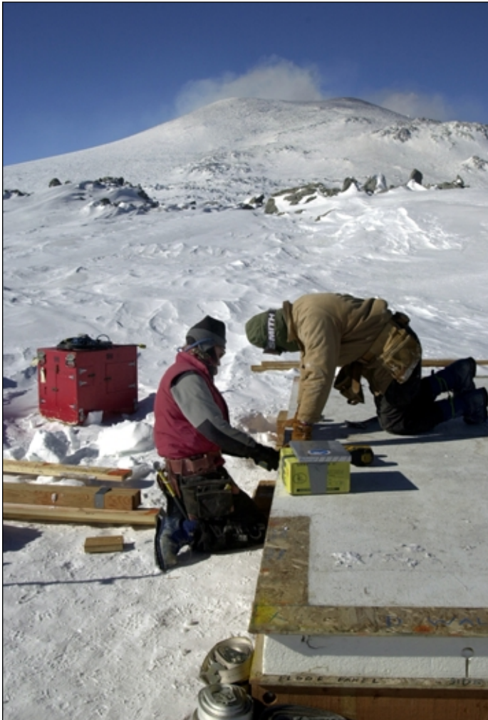
Eric "Homer" Holm, left, and Mark "Commander" Melcon install the insulated floor of a new building at Lower Erebus Hut, about 11,500 feet in elevation. The top of Mt. Erebus spews gas and vapor in the distance. The crew of three (including Bo Baumgartner, not pictured) spent several days acclimatizing at a lower point on the volcano before starting the high-altitude construction. Photo by Josh Landis.
