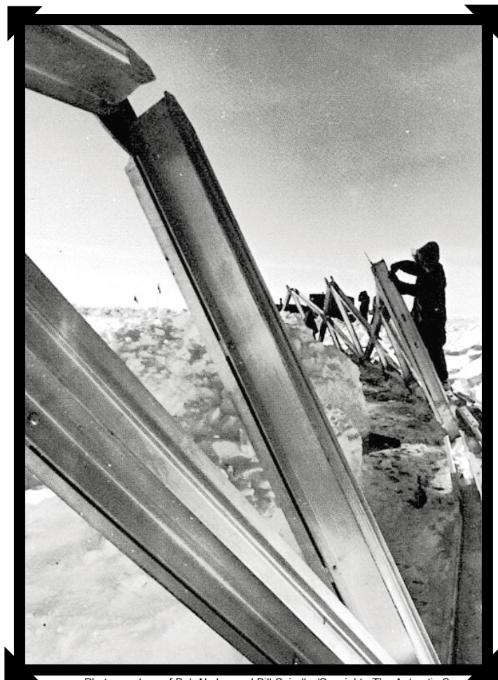
Photo courtesy of Bob Nyden and Bill Spindler/Special to The Antarctic Sun Seabees assemble the lower portion of the dome ring in 1972-73.
