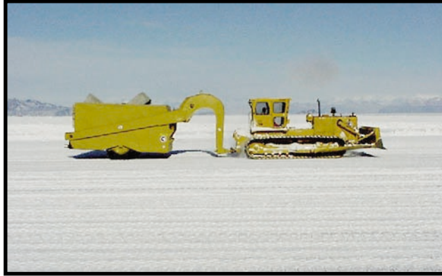
Photo by Gary Cardullo/Special to the Antarctic Sun A D-8 tractor tows a 100-ton roller, compacting the snow on Pegasus runway.
