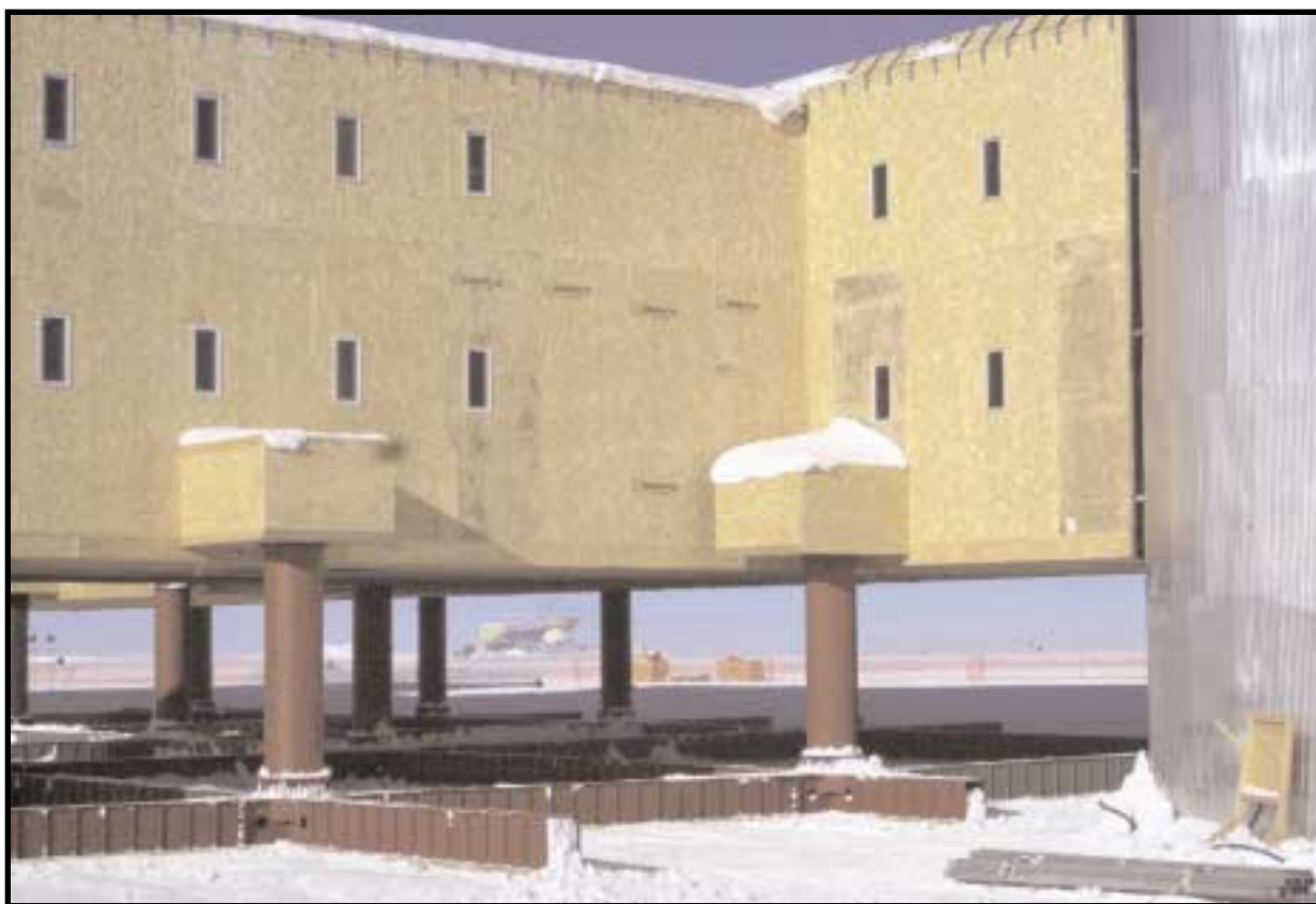
At left, the footings under the main section of the new station have been settling faster than the staircase tower. Below, workers jack up the station in increments to bring the sections level with each other.
