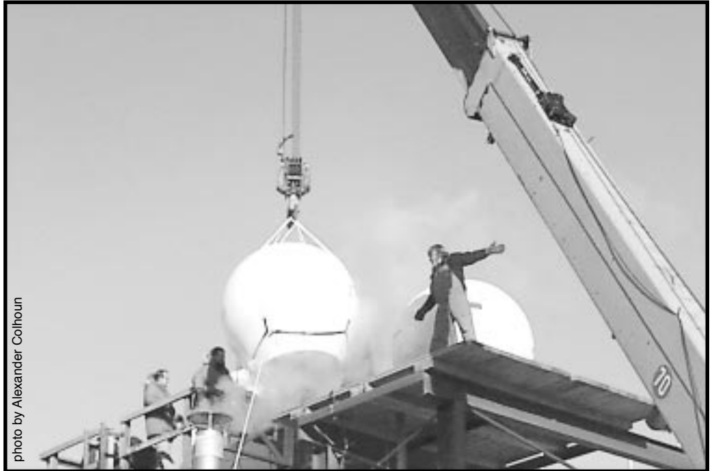
A new TERA SCAN satellite weather imagery system was installed in McMurdo last week. "It'll give weather forecasters and pilots better weather imagery between here and Lyttelton [New Zealand]," said Jim Johnson, assistant data systems manager in McMurdo.
