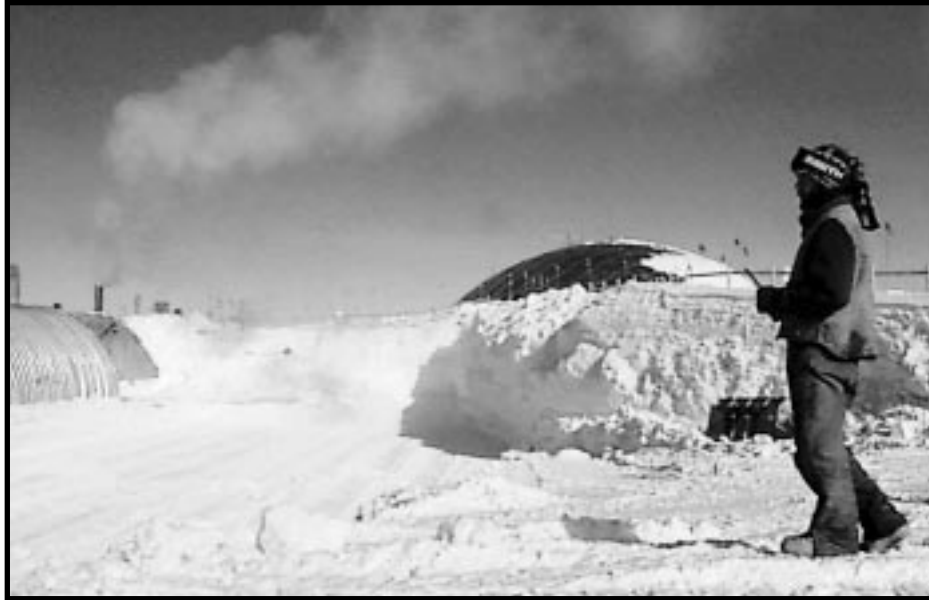
Carlton Walker, ASA Construction Supervisor, watches as D-7 bulldozers move thousands of pounds of snow to make room for a new 200-foot long, 64-foot wide, and 34-foot high garage arch at South Pole Station.
