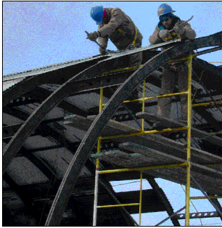
Charlie Blackmer, left, and Chris Craver strip metal sheets from the roof of the old playhouse. Photo by Jeff Inglis.
