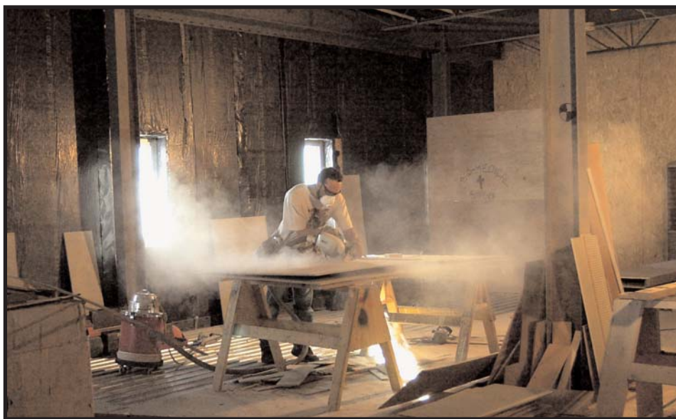
At left, a carpenter cuts plywood in one of the new sections of the South Pole station building. Above, a carpenter's apprentice puts finishing touches on the hall walls. An exterior view of the station is on page 1.
