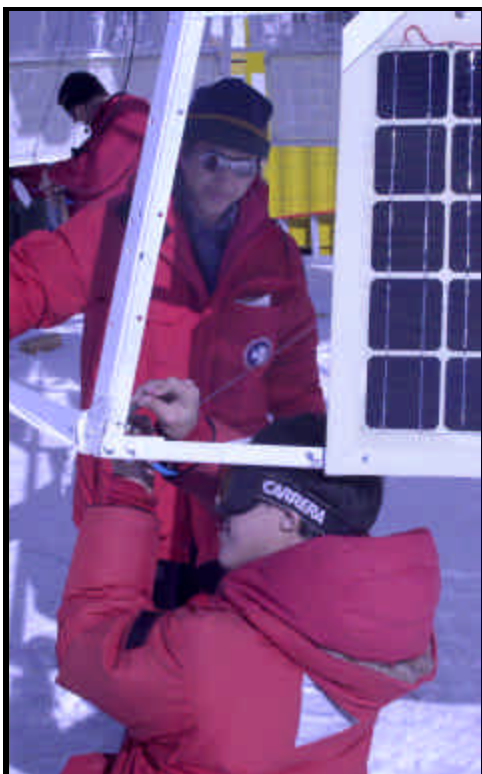
Photo by Brien Barnett / The Antarctic Sun Akira Yamamoto, the co-principal investigator with BESS, watches as Hideyuki Fume tapes a wire that stabilizes the solar panel array.
